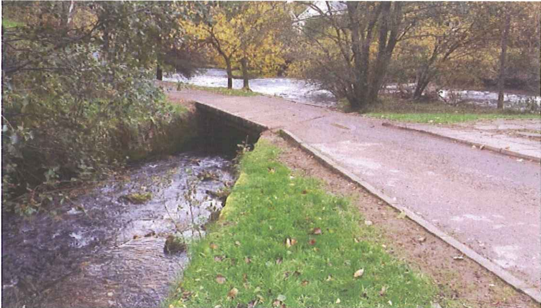
Photograph 9 – The bridge viewed from upstream
