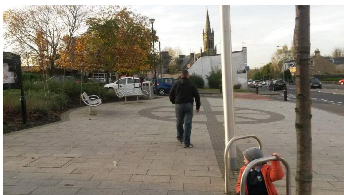
Concrete topped with granite aggregate
