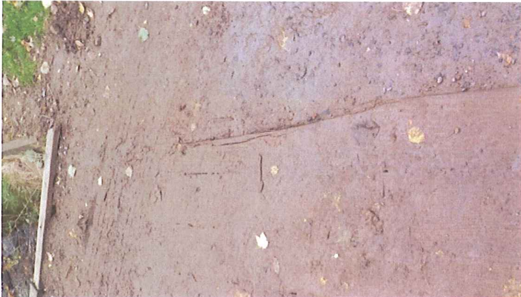
Photograph 15 – Condition of sleepers at point with road surface
