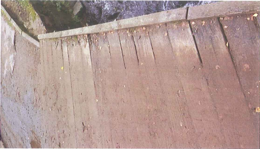
Photograph 14 – Downstream edge of the deck
