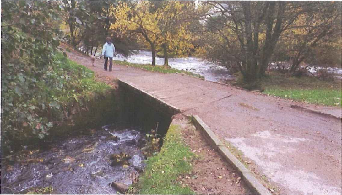
Photograph 8 – The bridge viewed from upstream
