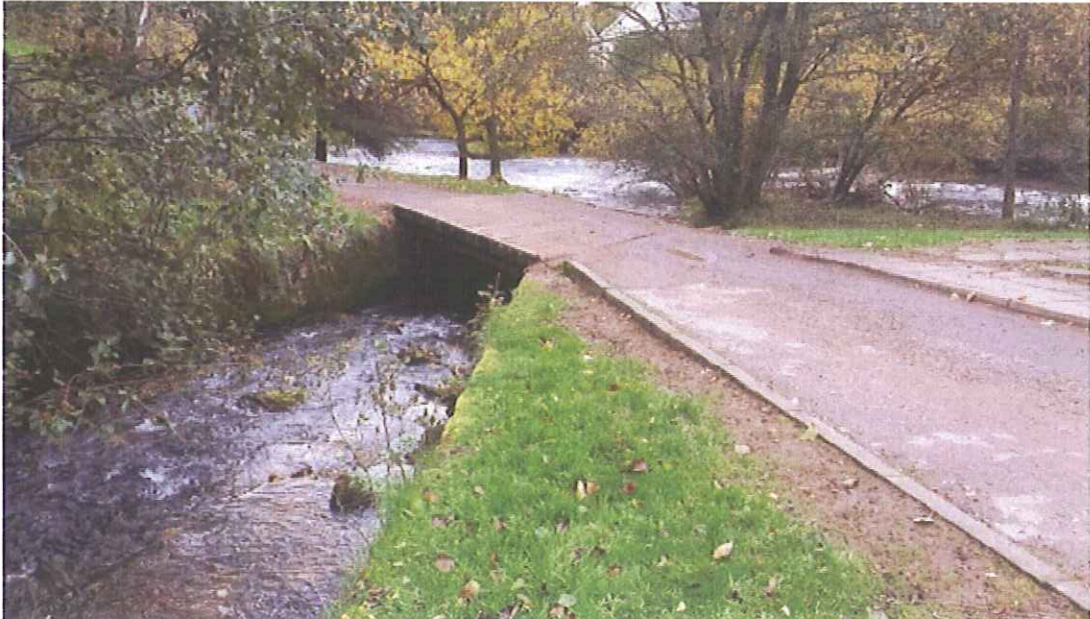
Photograph 9 – The bridge viewed from upstream
