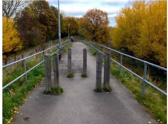
Looking from the bridge
