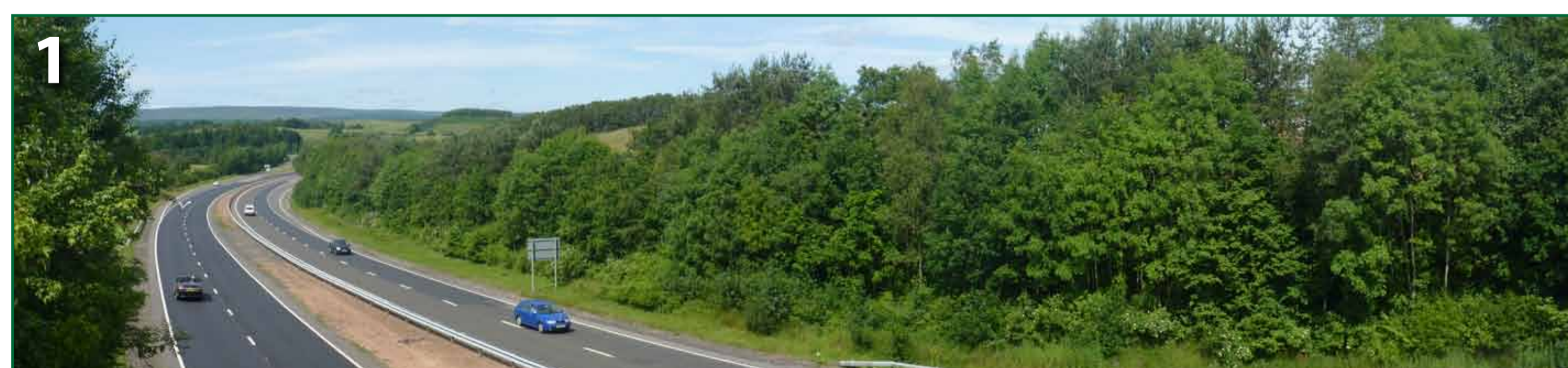
1 A9 forming Anchorscross site's western boundary
