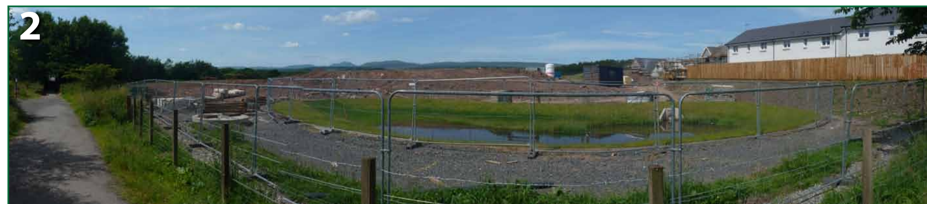
2 Anchorscross site situated next to new development along Old Doune Road
