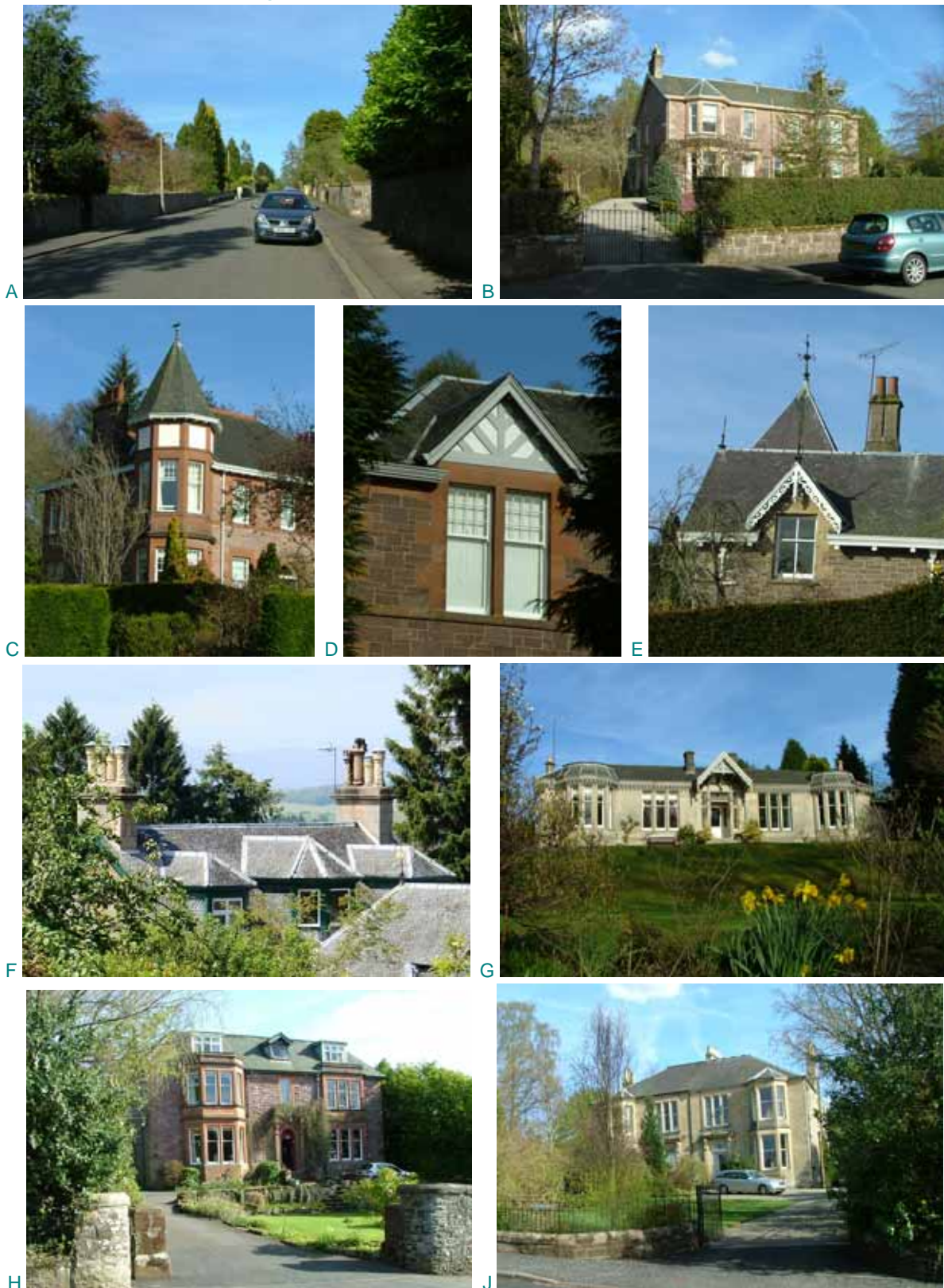
Fig 21A: Leewood Road looking NE, the road is fairly open with low stone walls, hedging and individual trees; B: St Margaret's Drive: a typical stone built semi-detached villa on raised garden ground behind low stone walls, hedging and ironwork gates; C – F: typical architectural details, in particular at roof level: turrets, timber gables, distinctive bargeboards, decorative slate-work and ornate chimney cans; G: Glenluss, an individual B-listed property on The Crescent; H: building types vary between asymmetrical detached villas (H) and symmetrical semi-detached houses (J).
