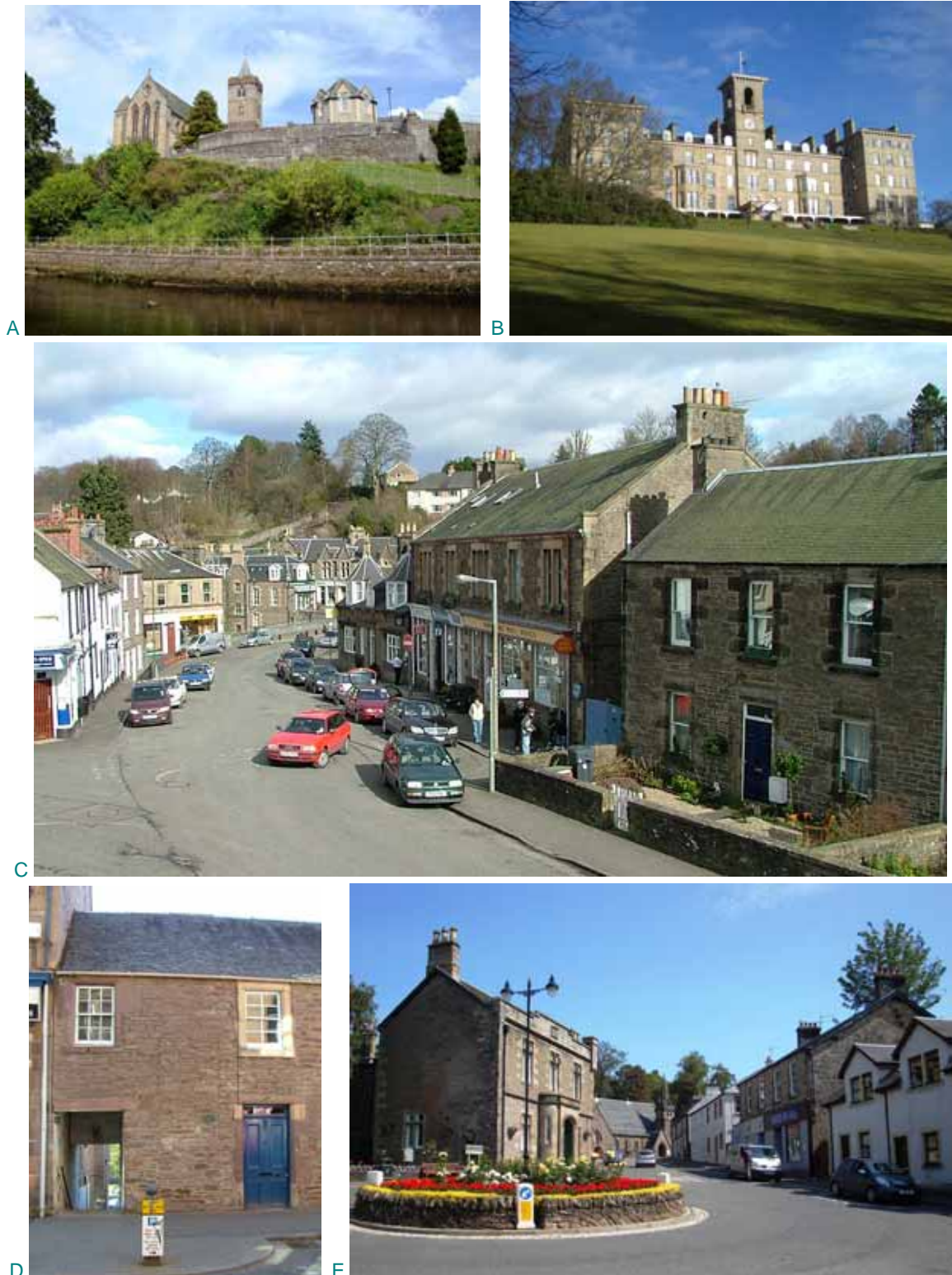
Fig 12A & B: Landmarks: A: Dunblane Cathedral viewed from the west bank of the Allan Water; B: the Dunblane Hydro, set in expansive landscaped grounds; C: view of Stirling Road, looking north-east from the footbridge over the railway. The broad sweeping road creates anticipation of the town and views to the High Street. Trees on Holme Hill and in private gardens behind the High Street and St Blane's House provide an important green backdrop and skyline feature; D & E: Street pattern: the old town retains the majority of its medieval street form with narrow lanes, pends (D), and winding roads such as the upper section of High Street (E).
