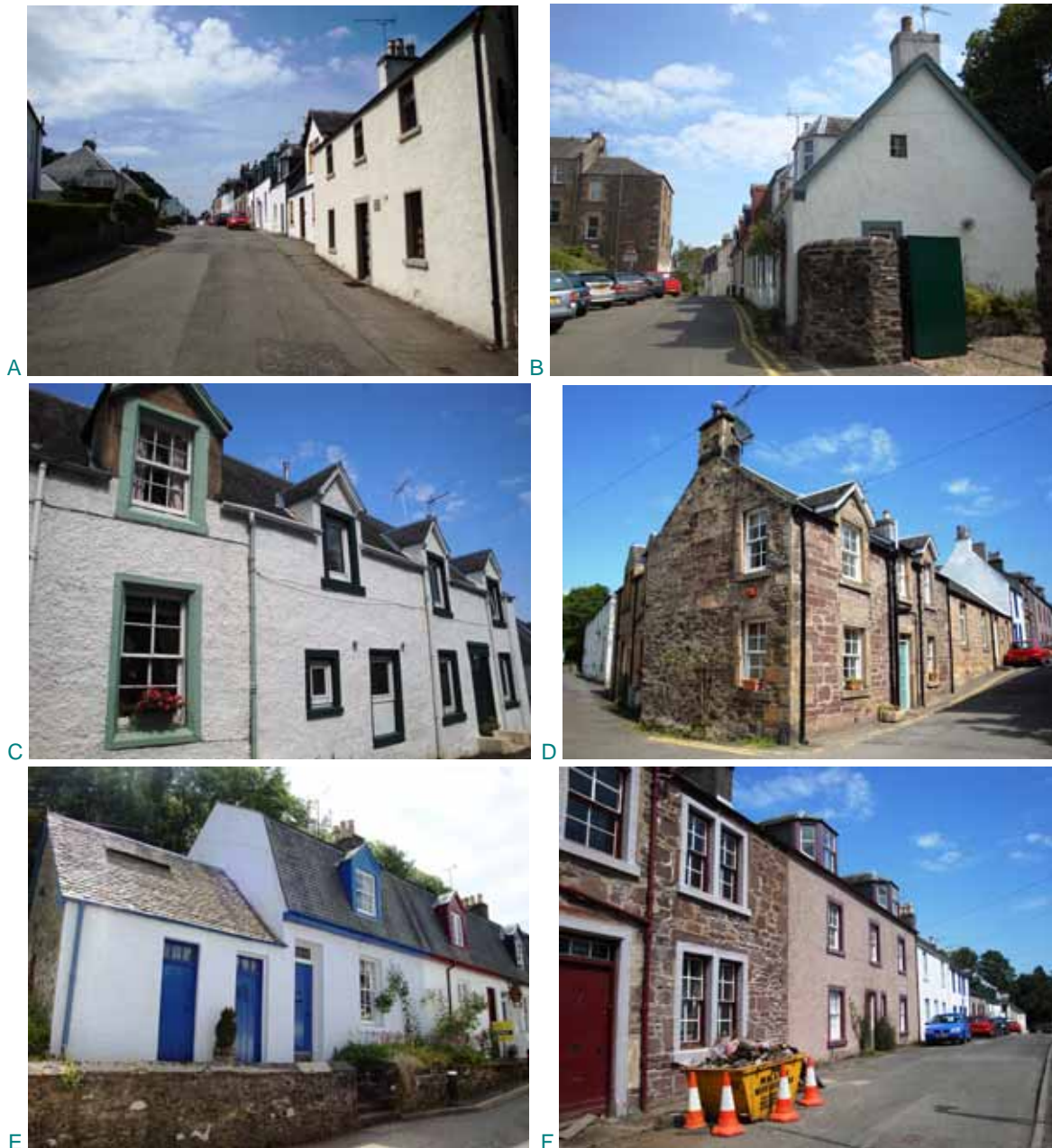
Fig 19A: Ramoyle looking west; B: Ramoyle looking east; C: dormers projecting through the eaves line are common on single storey properties, note the traditional windows on the house to the left which add character; D: Braeholm, a refined house which stands out on its corner site, original windows are a strong feature; E: single storey cottages with traditional timber doors; the later mansard roofs are not sympathetic, note low boundary walls and short front gardens in this location, and trees of Holme Hill forming an immediate backdrop; F: Airds and Ramoyle House (centre with canted dormers) are two good examples of the small 2-storey residences, both retain traditional windows and doors.
