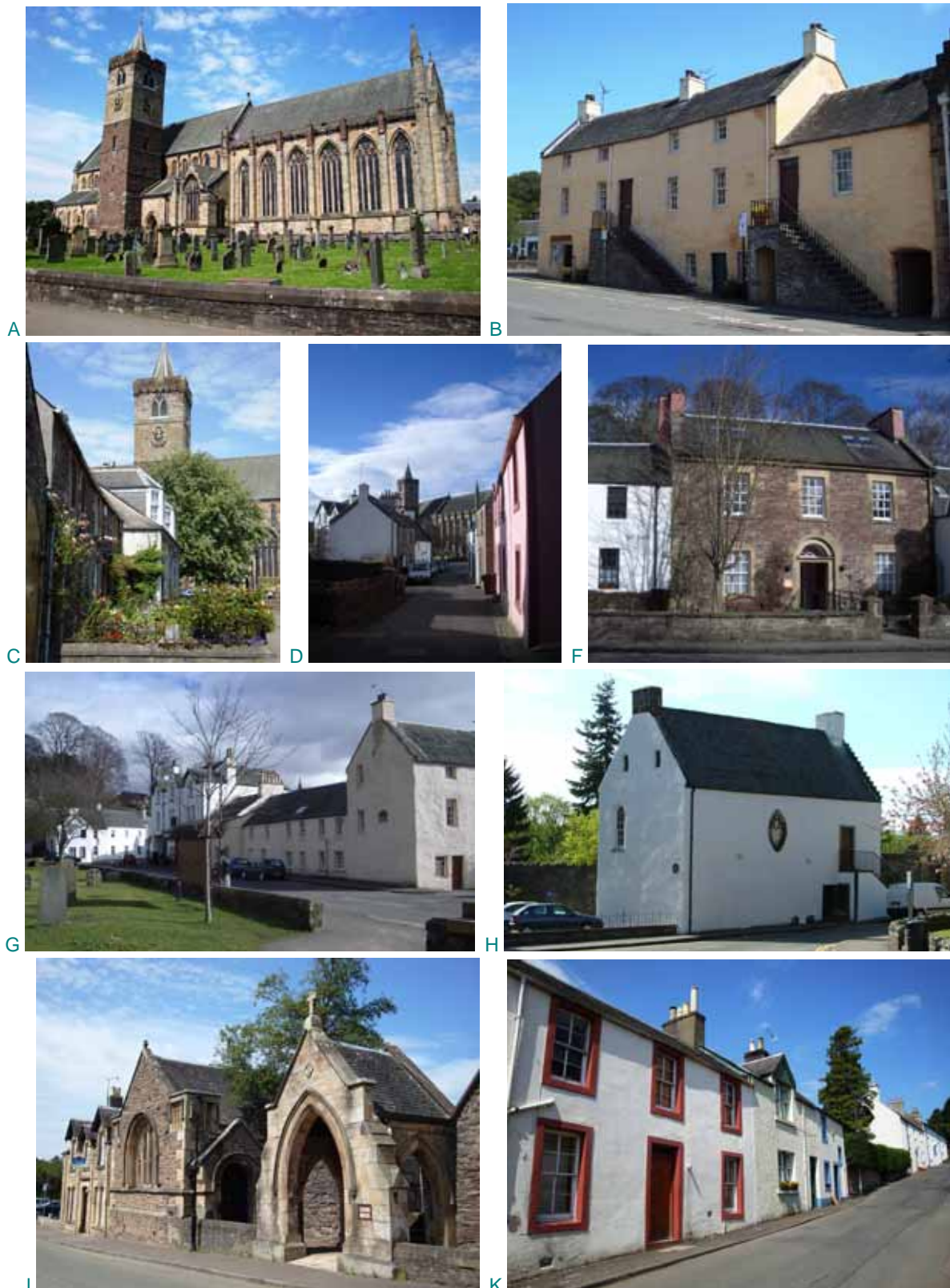
Fig 18A: Dunblane Cathedral; B: Dunblane Museum (the former Dean's manse) defines the corner of The Cross and Kirk Street; C: low cottages on The Cross form a picturesque setting for the cathedral; D: the twisting form of Sinclair Street creates anticipation as the cathedral comes into view; E: distinctive entrance to the Scottish Churches House; F: view of the south side of Kirk Street with Dunblane Museum occupying a significant section at The Cross and the 3-storey Tappit Hen beyond; G: Leighton Library at the foot of The Cross; H: Leighton House on the Haining; I: two important groupings of traditional properties on Braeport; Gigha is on the far left.
